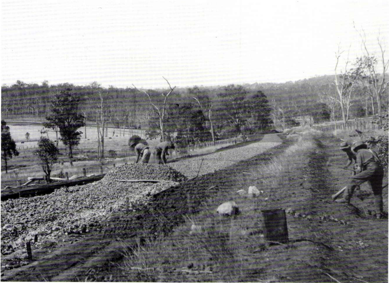
Roadworkers on Esk–Hampton Road, 29 April 1924.
