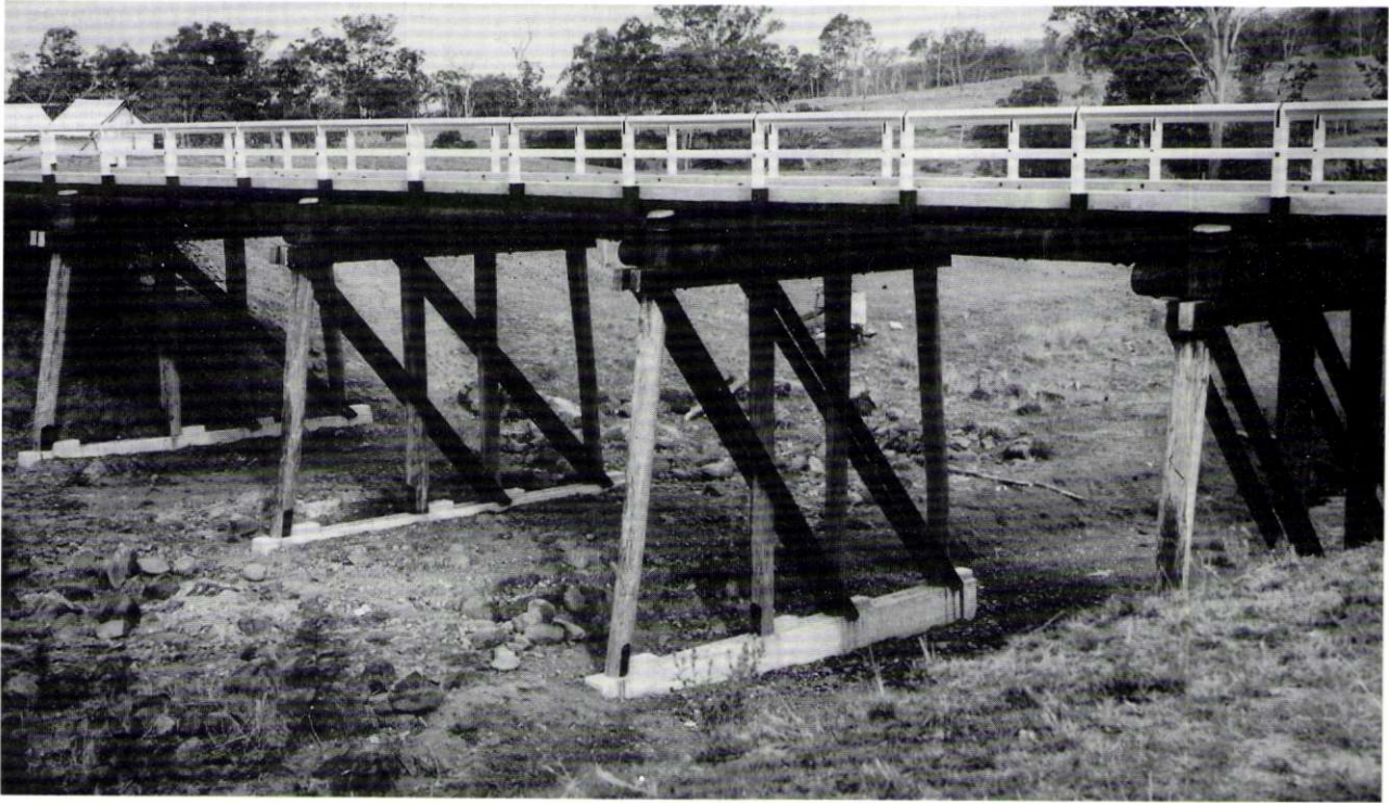
Bridge over Wallaby Creek on Brisbane Valley Highway. 1950s.
