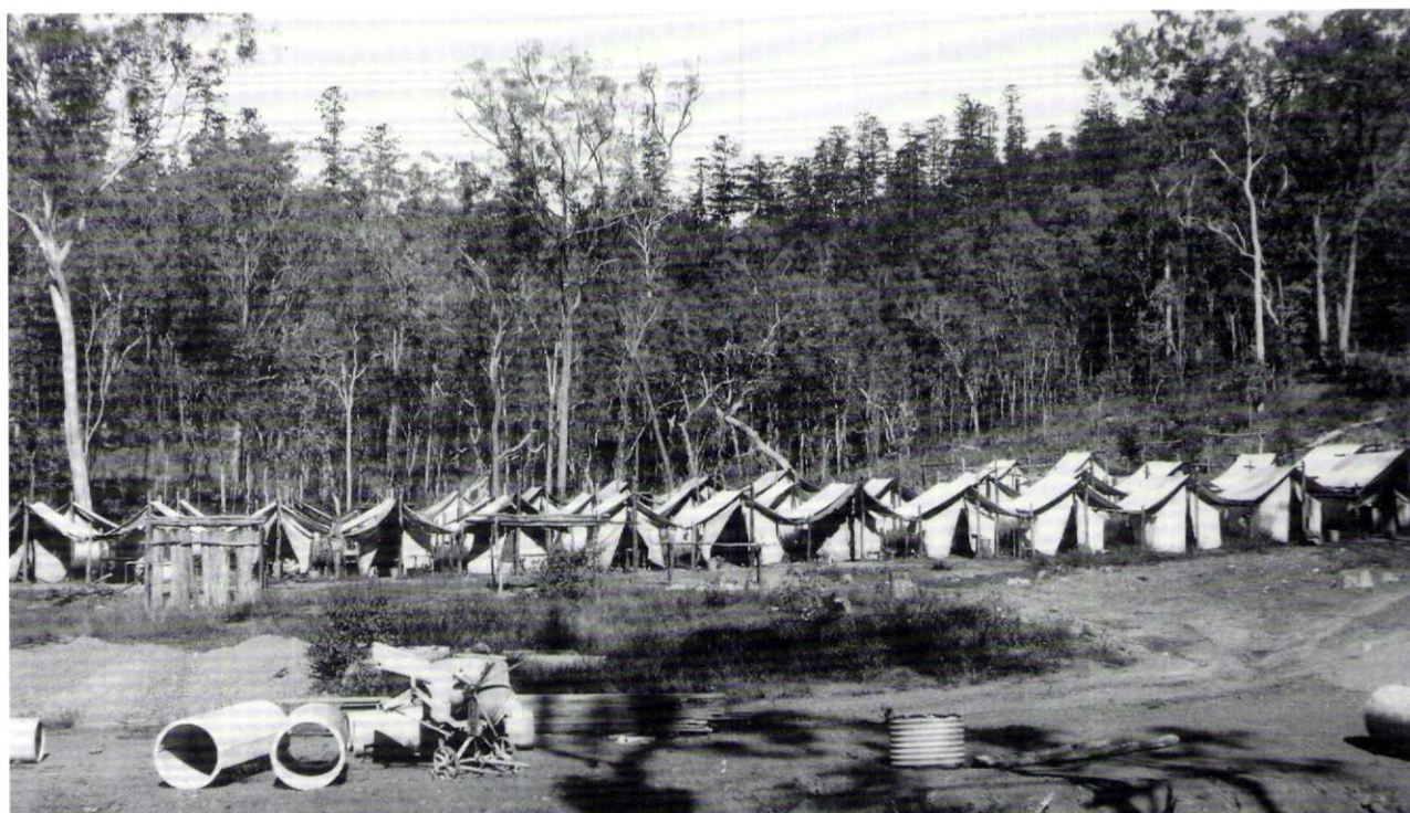
Construction workers' tents on Blackbutt Range. 1930s.
