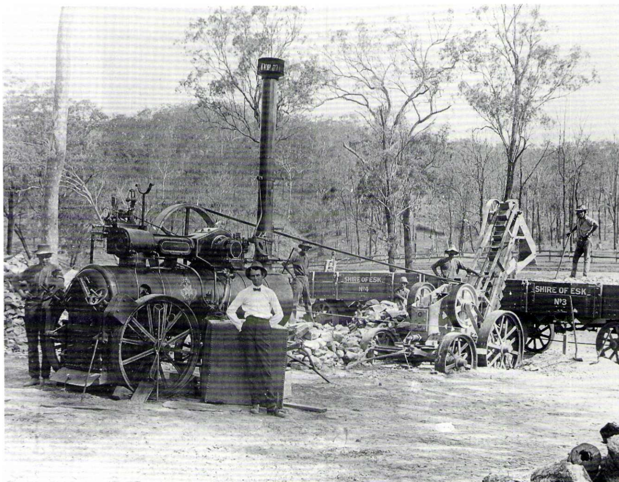
Engineer P.W. Hill in front of Esk Shire Council portable boiler and crushing plant. 1914.
