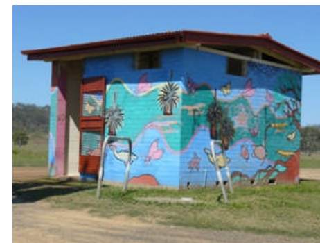
Photo 3: Photos of Twin Bridges Reserve
