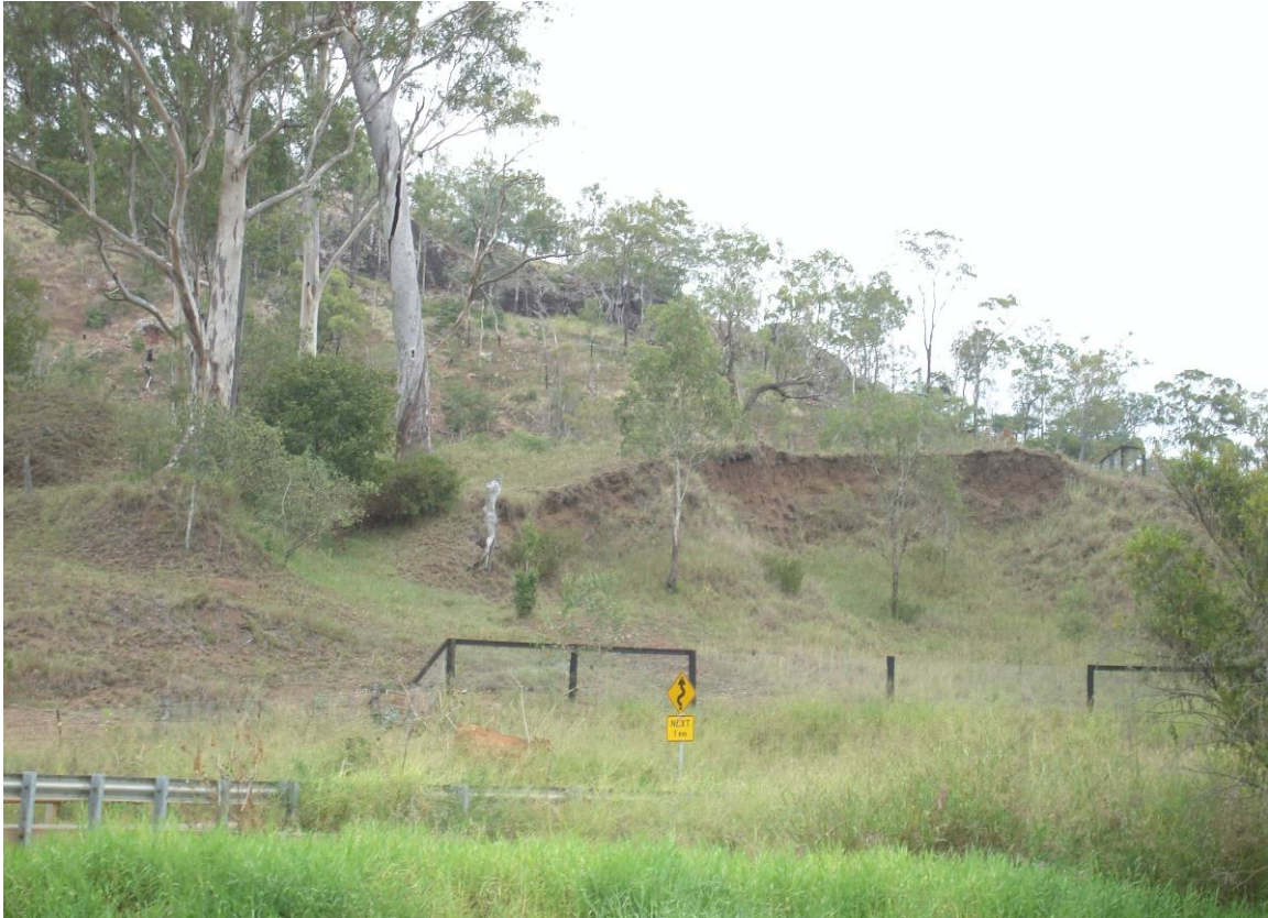
Plate P5: Hillslope Erosion Near Savage's Crossing.
