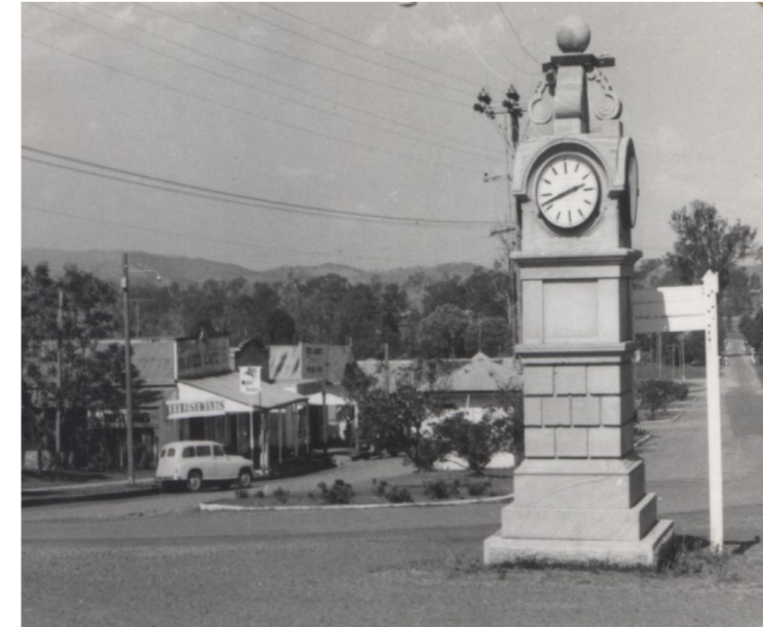
The William Butler Clock Tower looking East on William Street.
