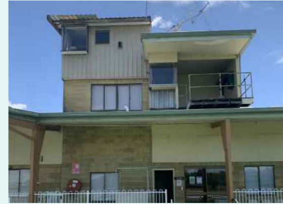
Race Caller Box and Viewing Tower - requires upgrade and improved access
