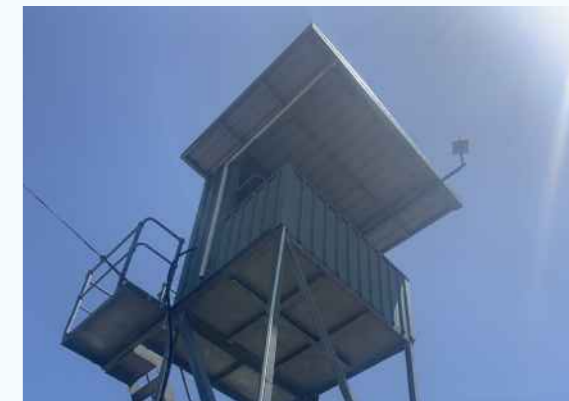
Race Viewing Towers - located at key locations on perimeter of race track and currently fit for purpose
