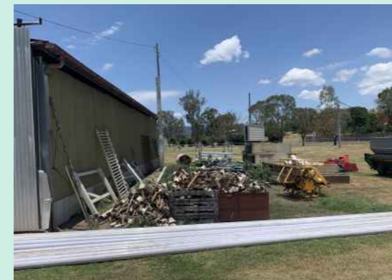
Race Club maintenance equipment stored externally - insufficient storage and poor aesthetic appeal
