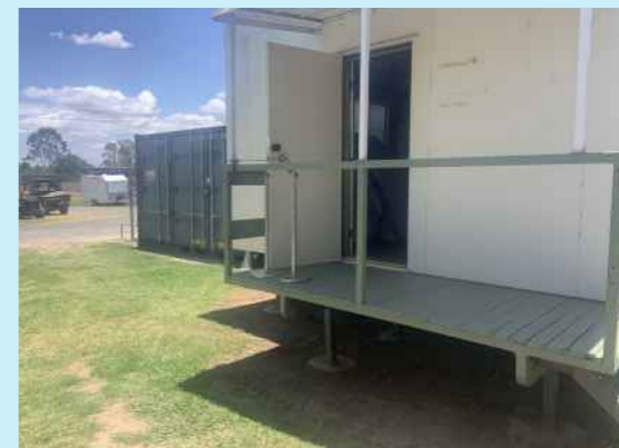
Race Club Storage - poorly located and insufficiently sized
