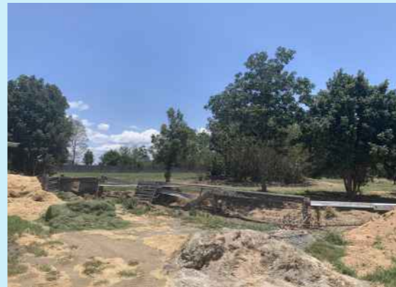
Deco Pits - will require relocation due to proposed new road alignment
