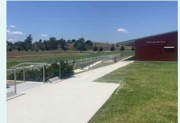
Trackside Pavilion - newly constructed and fit for purpose
