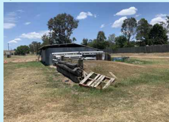
Loading Ramp and Pony Club Storage Shed - no longer required in this location and not fit for purpose
