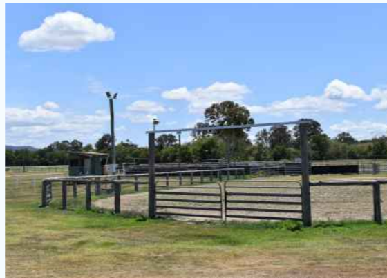
Rodeo Arena - requires lighting installation and fencing upgrade in the future
