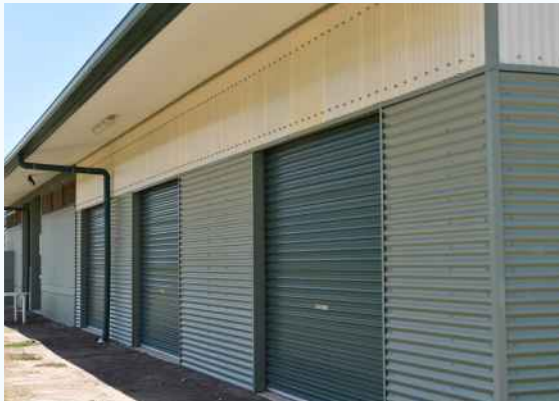
Ken & Mary Nunn Pavilion (Storage Bays) - newly constructed and fit for purpose
