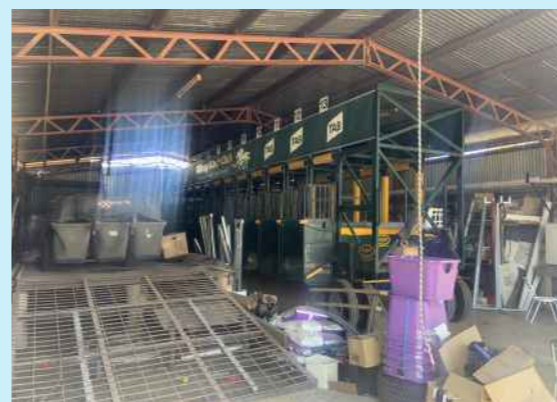
Race Club Maintenance Shed & Storage - insufficient size
