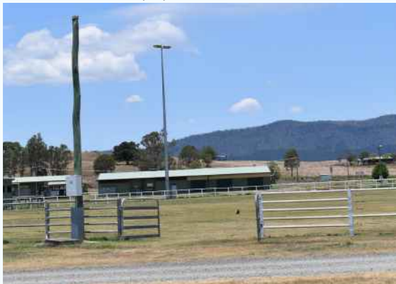
Main arena - large open space with partial lighting, requires additional lighting
