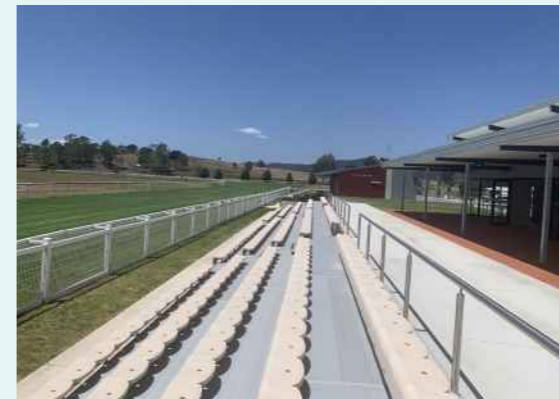
Grand stand seating - newly constructed and requires shade cover
