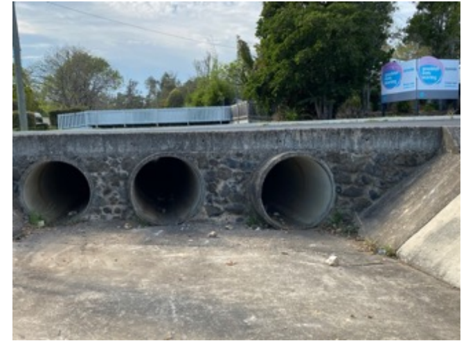
Drain along Burns Street
