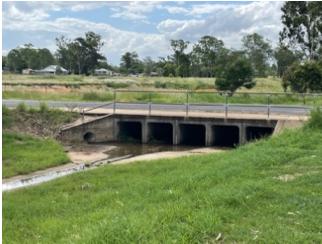
Drain along Banks Creek Road
