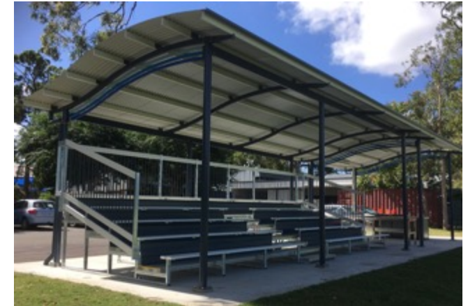
Figure 38: Covered spectator grandstand (Source: Outdoor Design, 2017)
