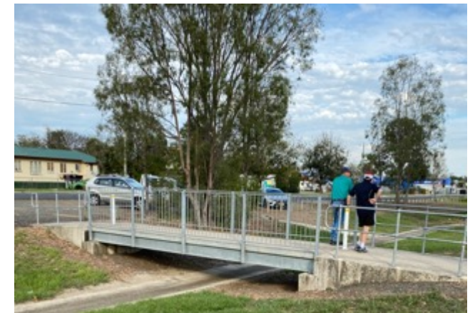
Pedestrian Access Bridge at Stumer Park
