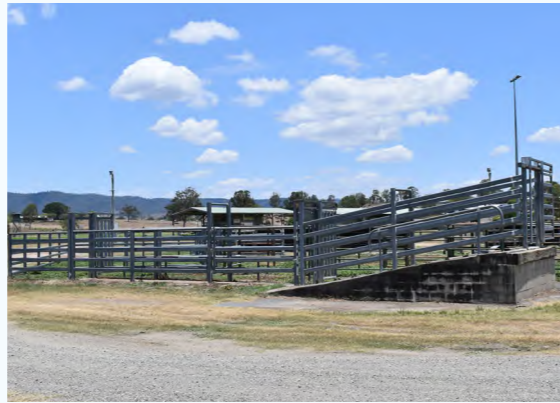
Cattle Yards & Loading Ramps - currently fit for purpose will require renewal in the future
