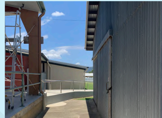
Limited integration of existing buildings with newly constructed buildings
