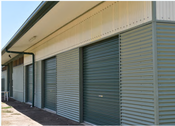
Nunn Pavilion (Storage Bays) - newly constructed and fit for purpose
