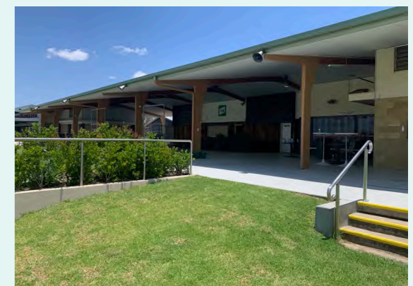
Main race club building - requires reconfiguration and expansion
