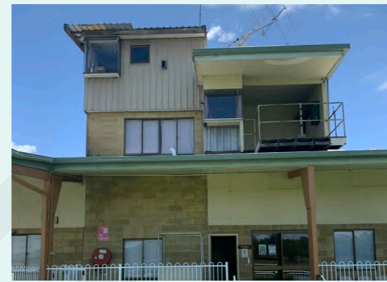
Race Caller Box and Viewing Tower - requires upgrade and improved access
