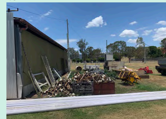
Race Club maintenance equipment stored externally - insufficient storage and poor aesthetic appeal
