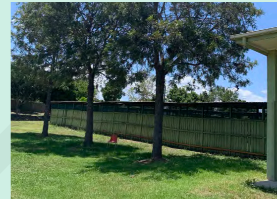
Rear of Tie Up Stalls - disconnected to ancillary elements
