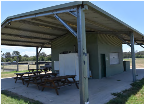
Nunn Pavilion (canteen/bar) - newly constructed with additional covered seating area required
