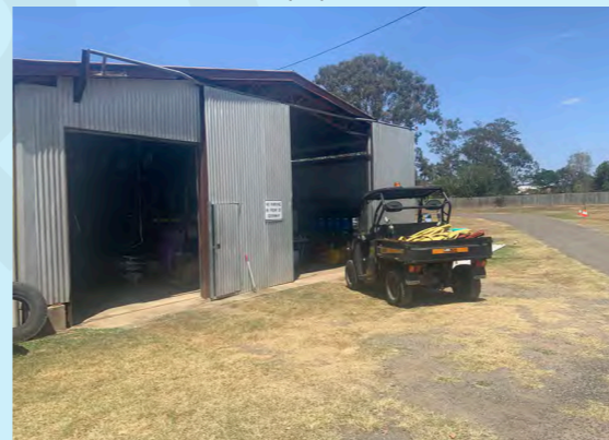
Race Club Maintenance Storage Shed - poorly located and insufficient size to accommodate all infrastructure
