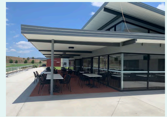
Dining/Food Pavilion - newly constructed and fit for purpose
