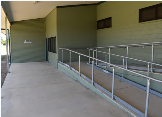
Nunn Pavilion (Toilets and Showers) - newly constructed and fit for purpose
