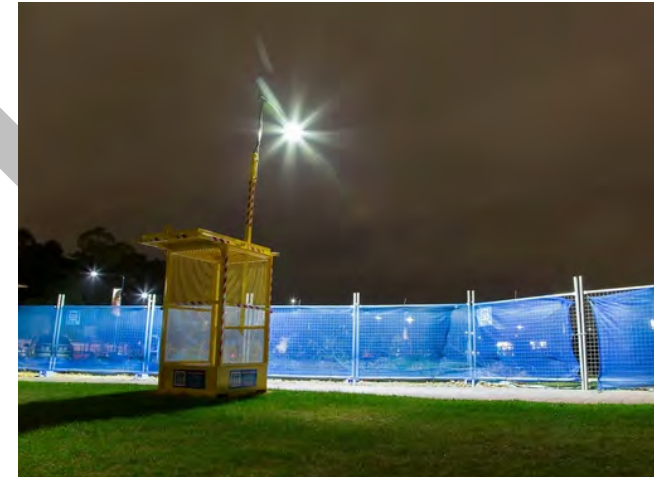
Figure 24: Arena lighting (Source: Google, 2021)
