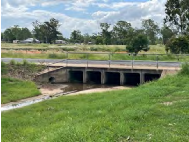
Drain along Banks Creek Road Drain adjacent to main entrance
