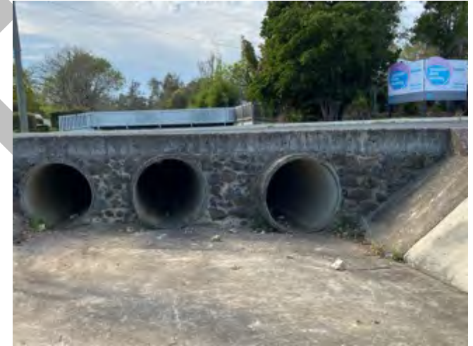
Drain along Burns Street
