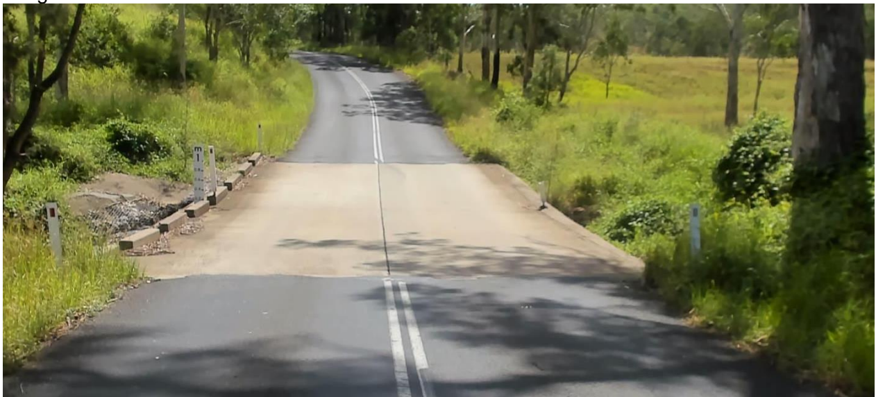
Gregors Creek Road - Ch9200 to Ch9370
