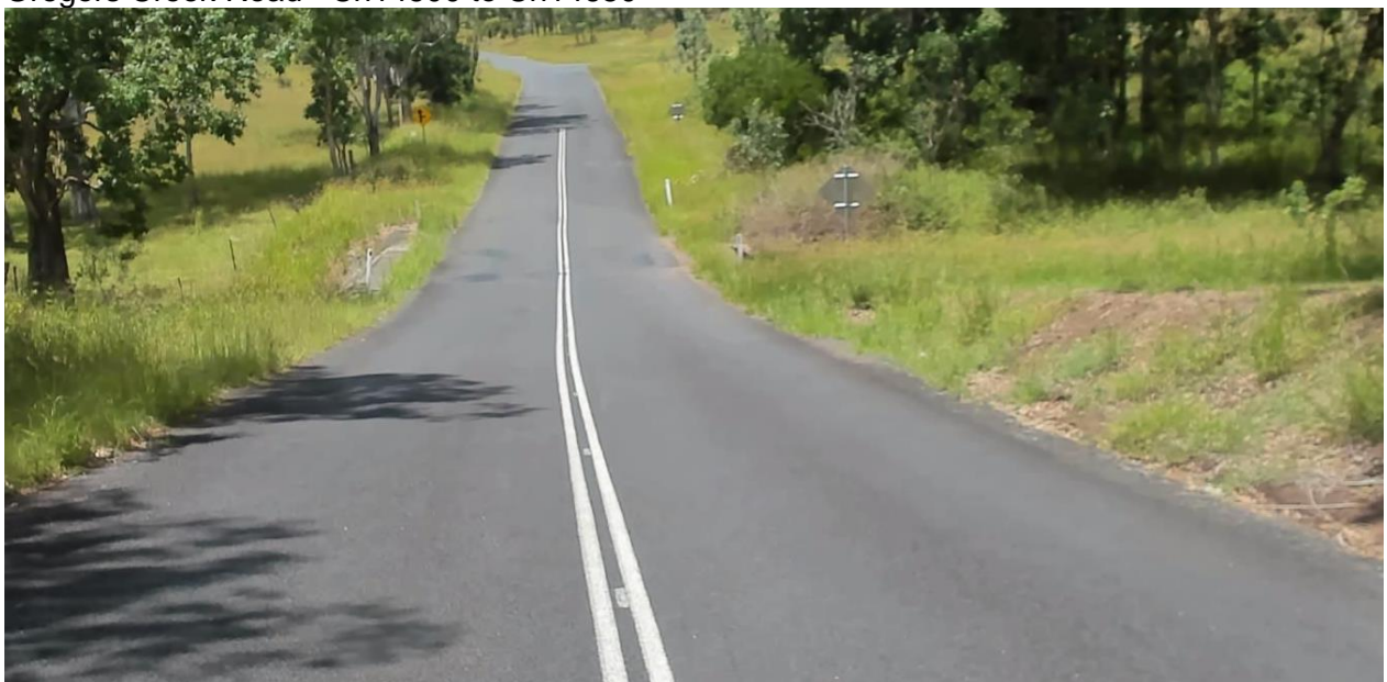
Gregors Creek Road - Ch14500 to Ch14680
