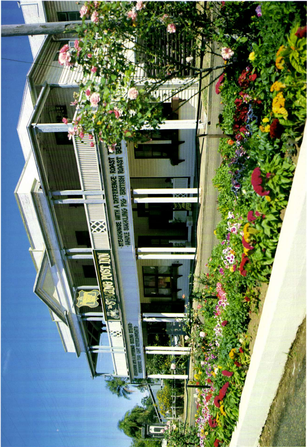
Staging Post Inn formerly Hotel Metropole and Ipswich Street flower gardens, Esk. 1987.
