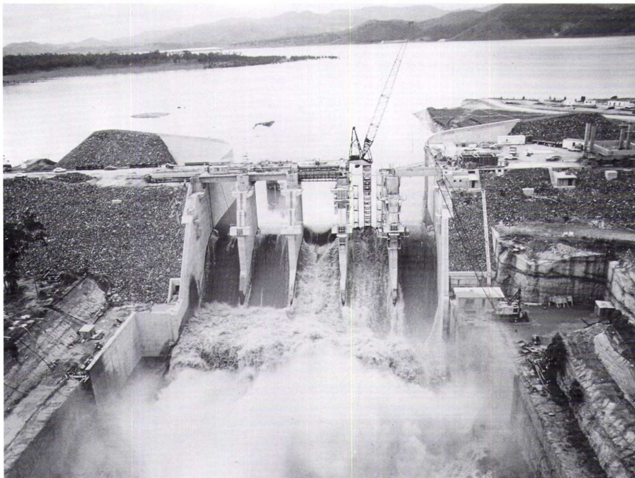
Wivenhoe Dam flooding during construction in 1983.
