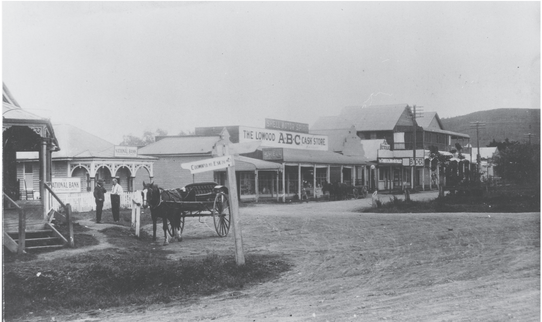
Main street of Lowood (Railway Street) in 1929, showing the heritage-listed former bank building to the left of the image. Image: State Library of Queensland
